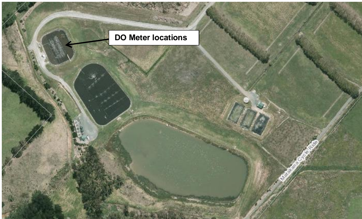
Figure 2 The location of two autonomous DO meters in the WWTP aeration pond
